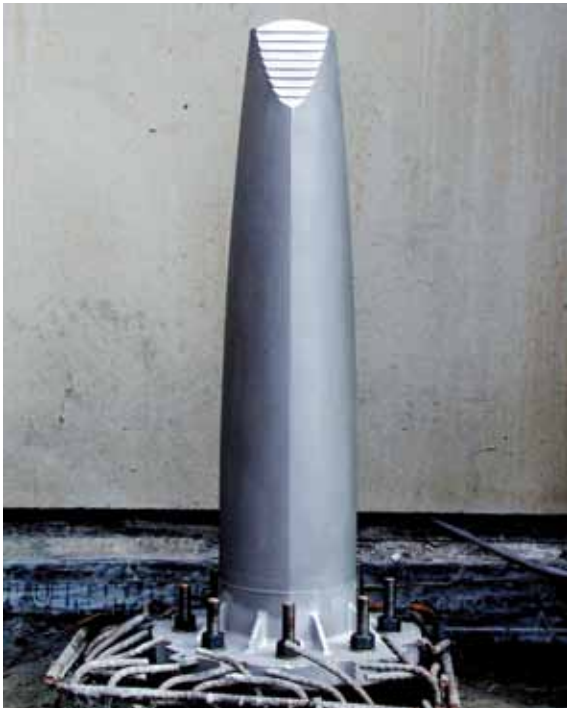
Fig. 1. Custom anti-ram bollard designed by Rick Reeder, fitted in reinforced concrete
