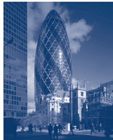
The impressive Swiss Re building is the fifth tallest in London and has won many architectural awards.
